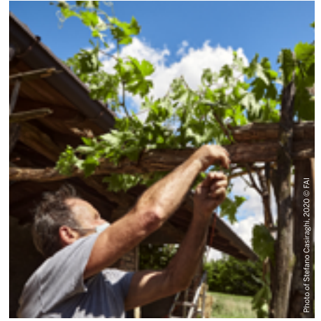
The initial maintenance works on the pergola
